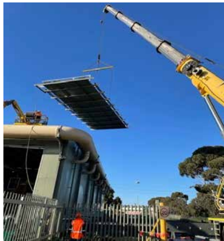
Roof replacement commenced July 2022
