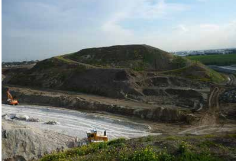
FIG 20 WESTERN LAND RECLAMATION SITE
