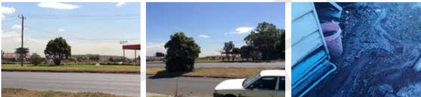
Figure 3 Stockpiles visible from Geelong Rd and dirt accumulating around the house
