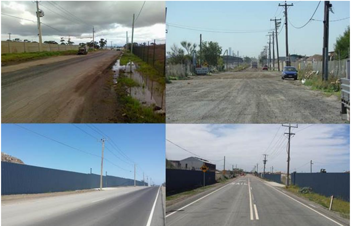
Figure 5. Jones and Bunting Rd – before and after sealing in November 2015
