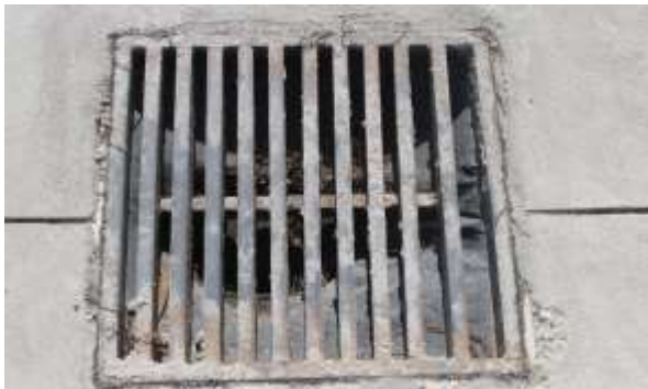
Installing filters on stormwater drains to eliminate contaminants from entering our waterways
