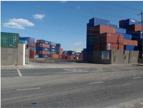
Figure 1 Site improvements at Rocke Brothers – before and after images
