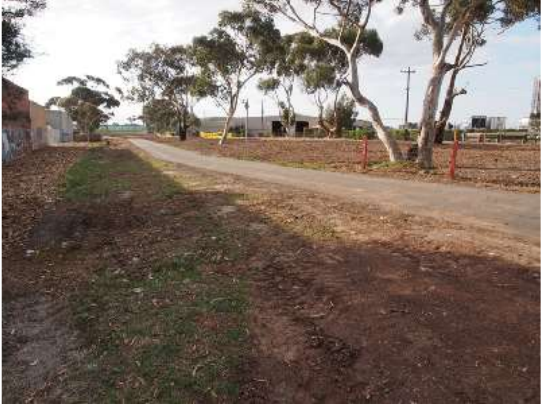
Trail site preparation including mulching
