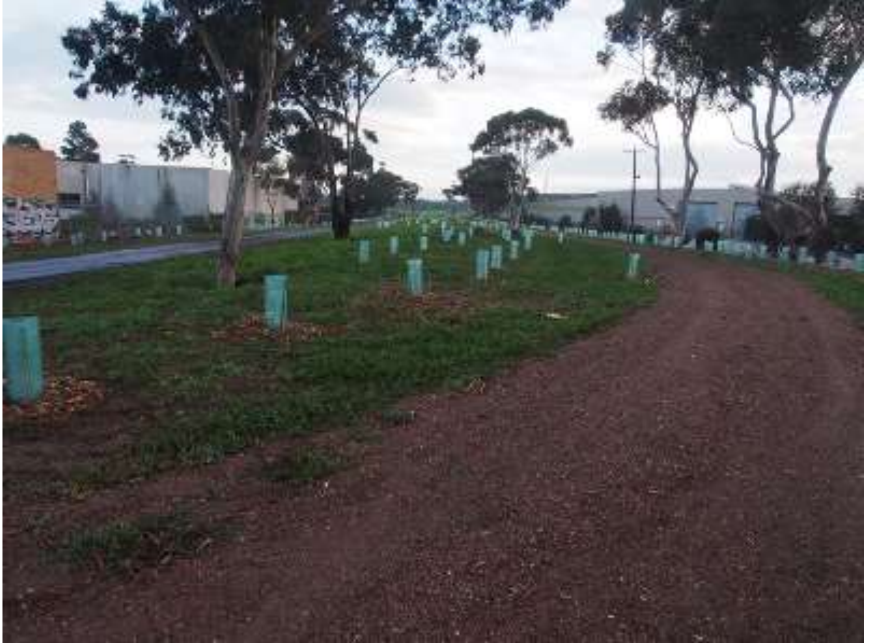
Planting commences along Federation Trail.
