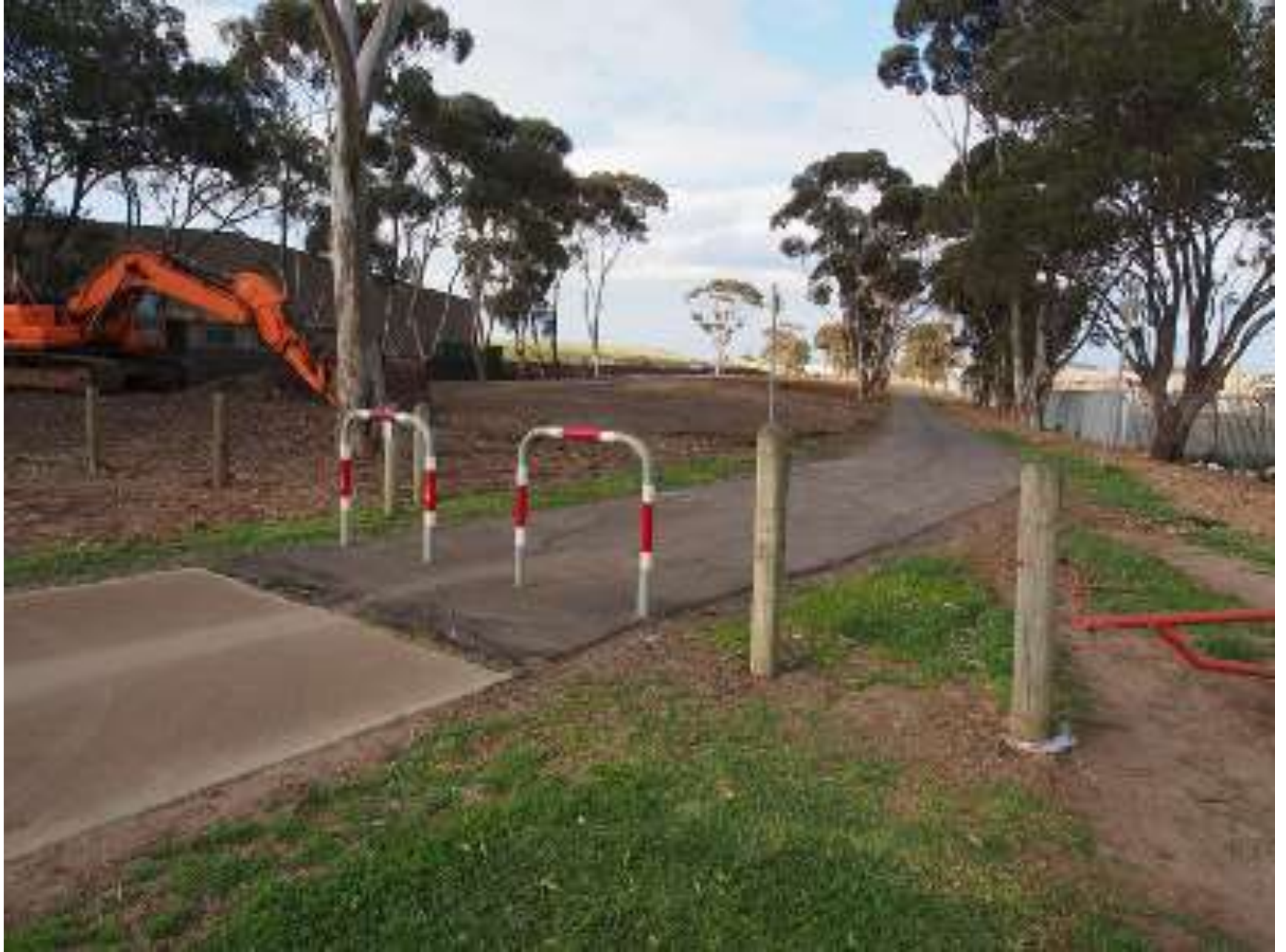
Trail site preparation including massive earth works
