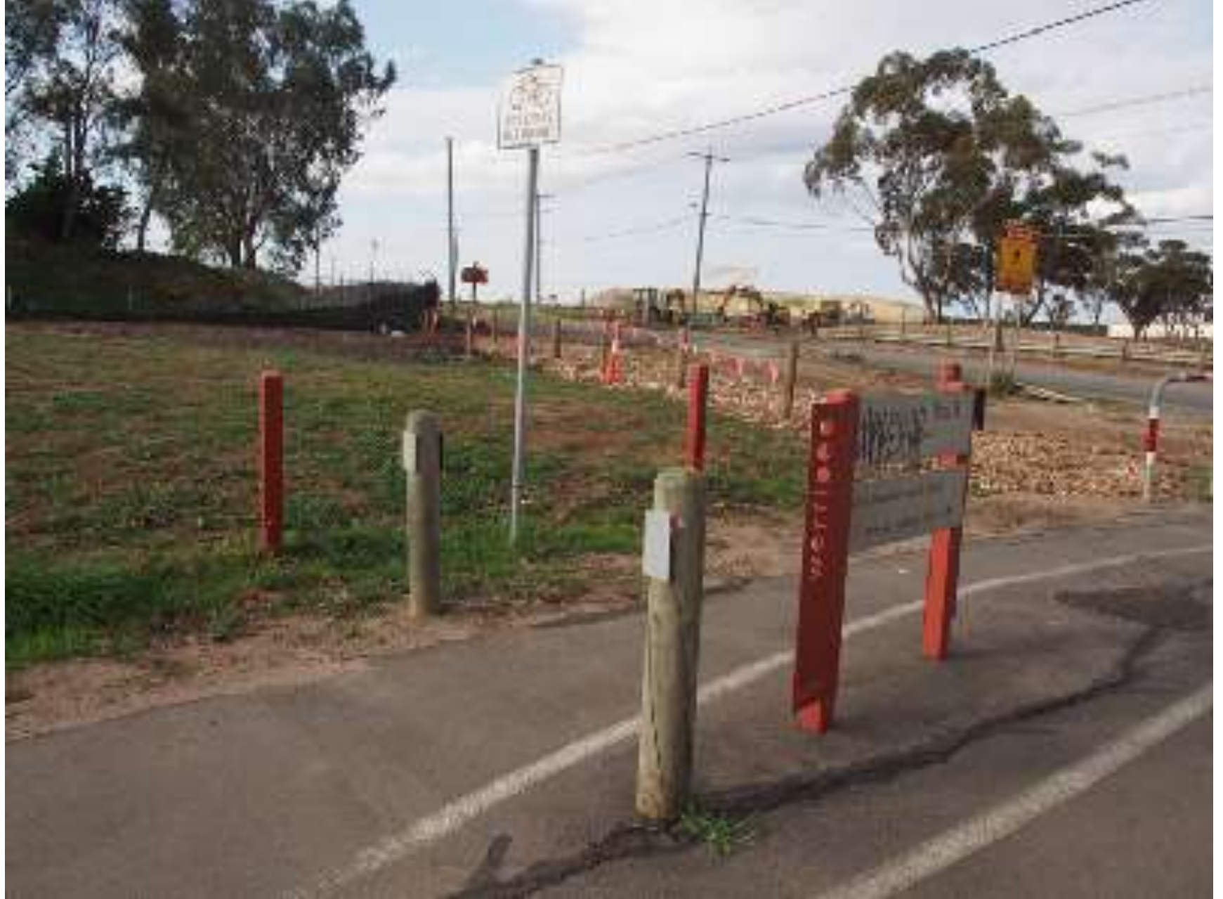
Trail site preparation including mulching
