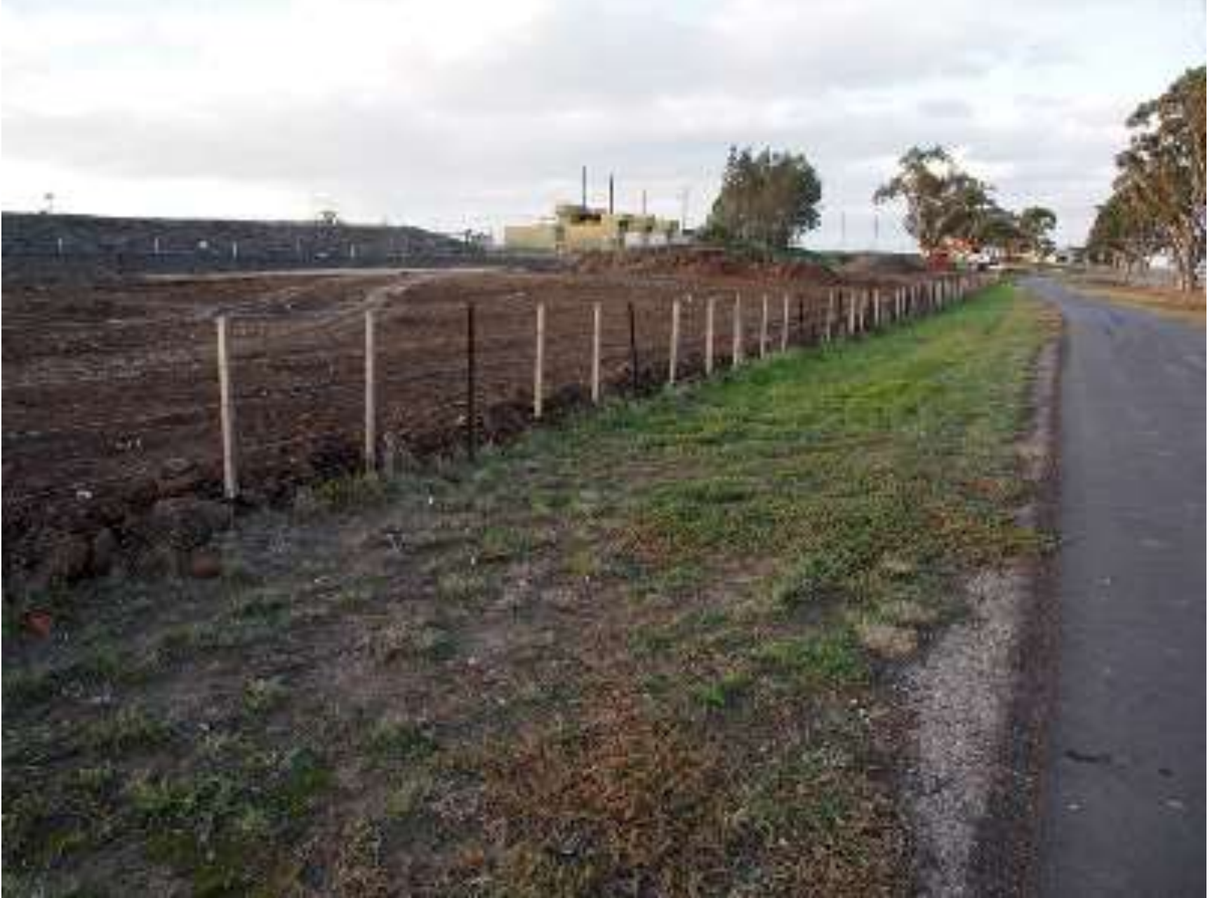
Trail site preparation including massive earth works
