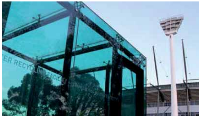
Yarra Park Water Recycling at MCG
