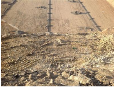
Landfill C4 capped
