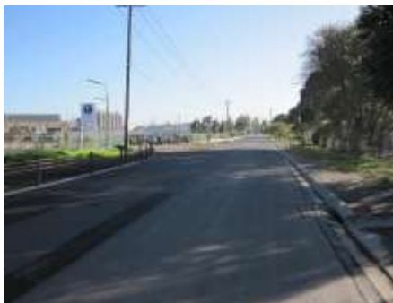
Slides 8 & 9 Wire barrier and steel barrier near Tasman Logistics entrance.
