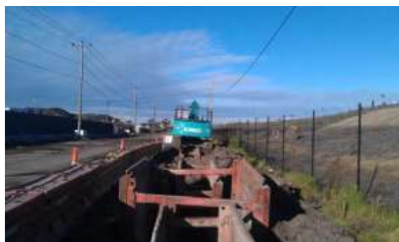
Drainage works in Jones Road
