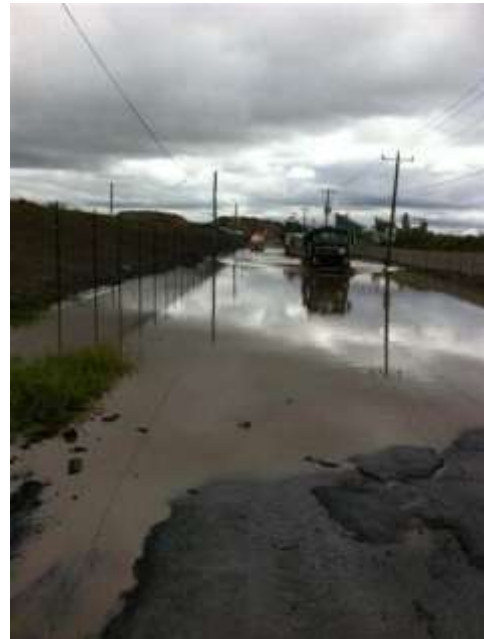
Fig 10 Jones Road before drainage works
