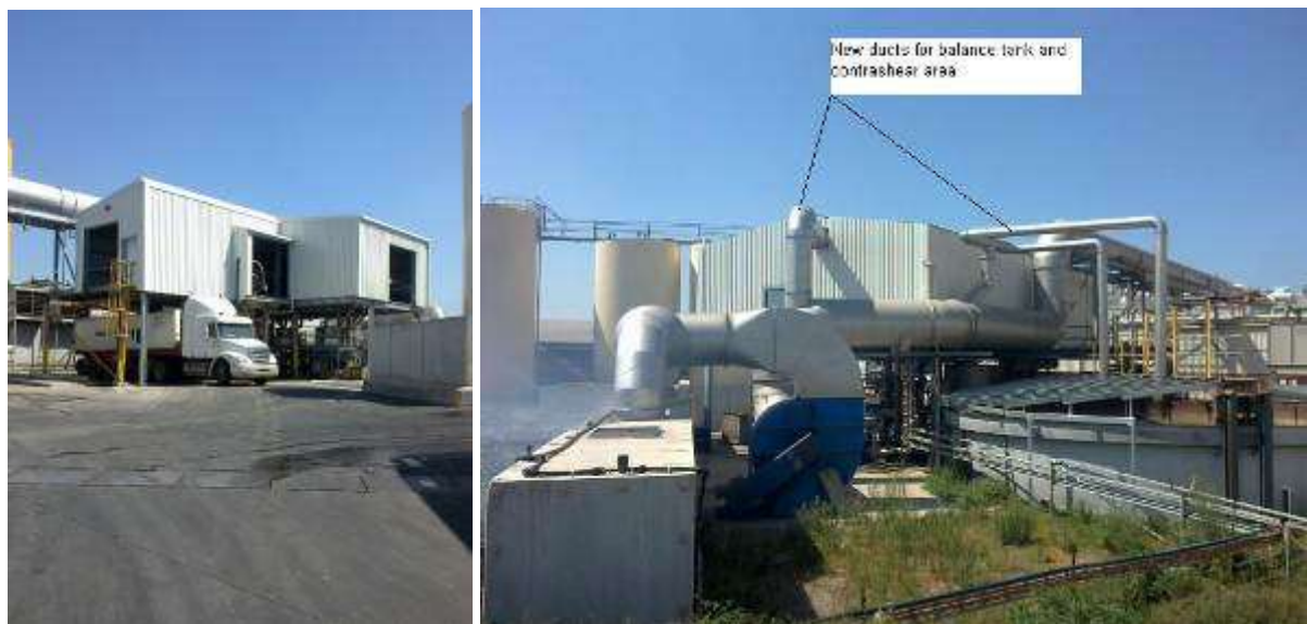
New building housing the first part of our waste water treatment plant
