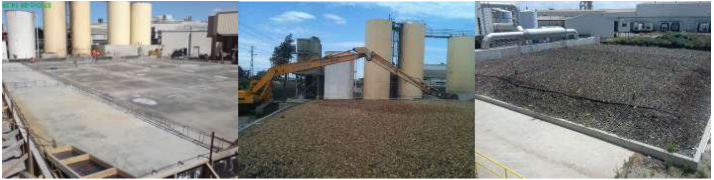
Biofilter foundation being laid October 2009
