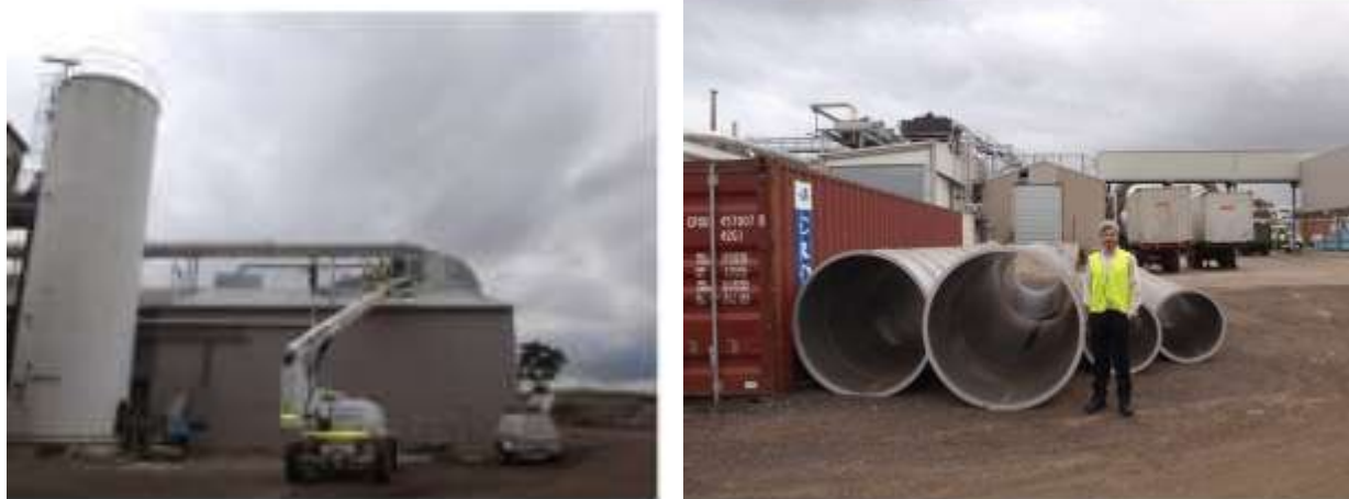
Fig 24 Slides 7 & 8 Improvements to ducting at ATP, ducting pipes.
